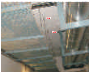
Cable Tray & Air Duct
