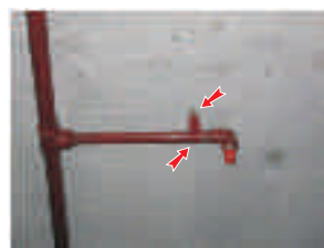
Fire Fighting Sprinkler
