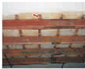
Fixing of Earthquake resistant beams
